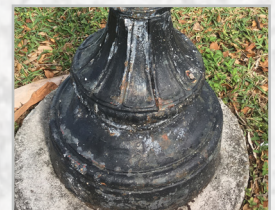
Metal Pole Corroding
