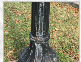
Metal Pole Corroding
