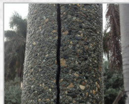
Concrete Pole Cracking
