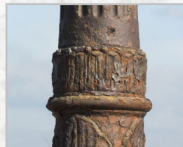
Metal Pole Rusting
