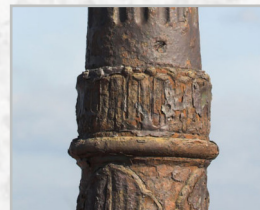
Steel Pole Rusting
