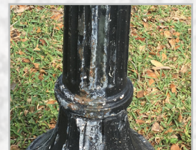
Aluminum Pole Corroding
