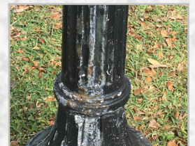
Aluminum Pole Corroding
